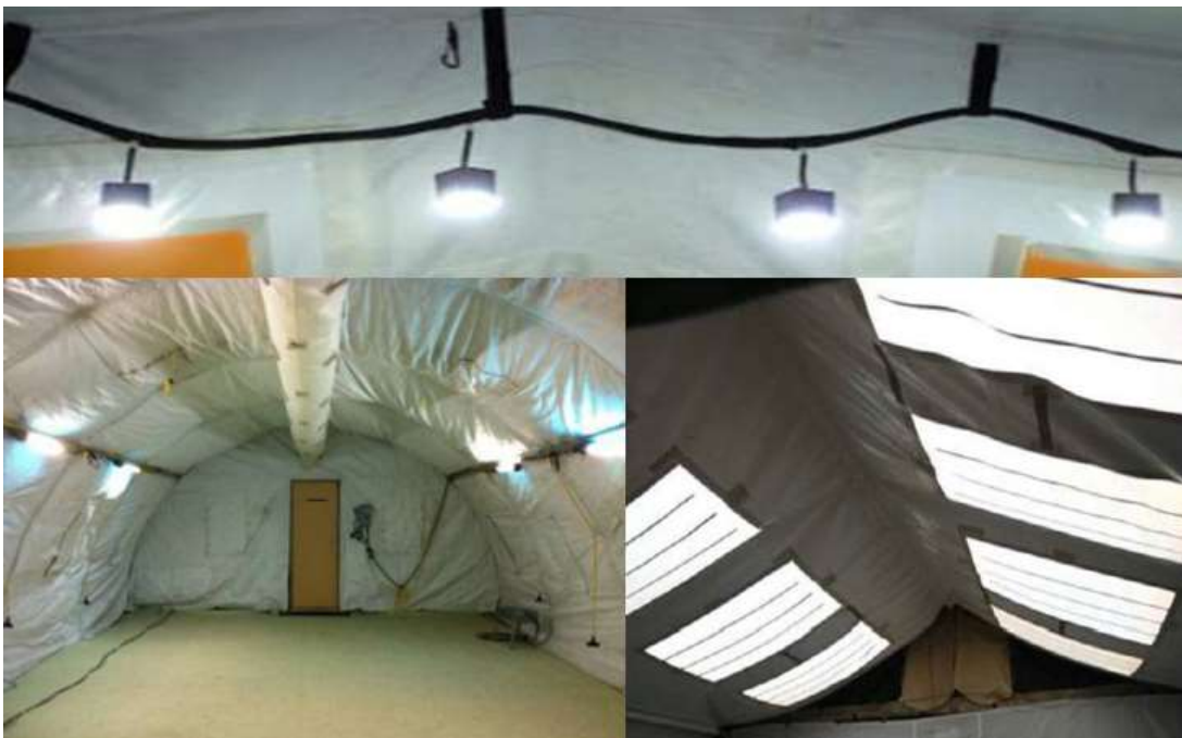
Figure 2. Various light sources for tents. LED (top), fluorescent tubes (left), Electroluminescence (right) [23].
