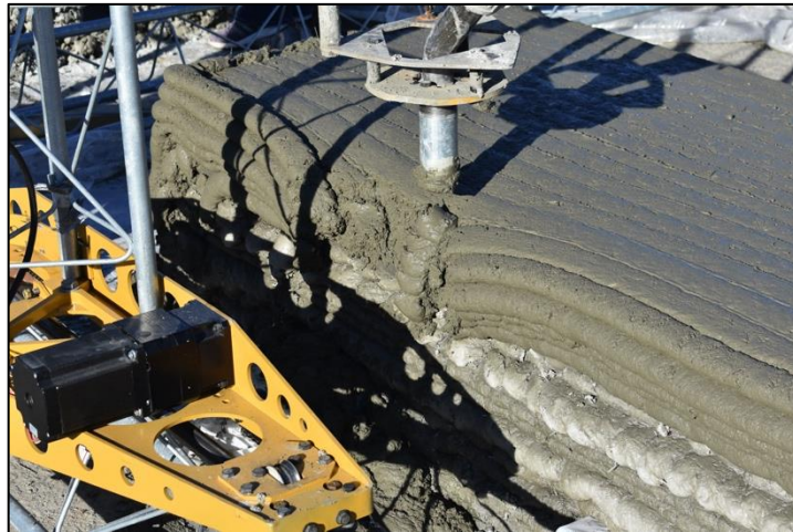
Figure 13. Material Collapse Under Self-Weight.
