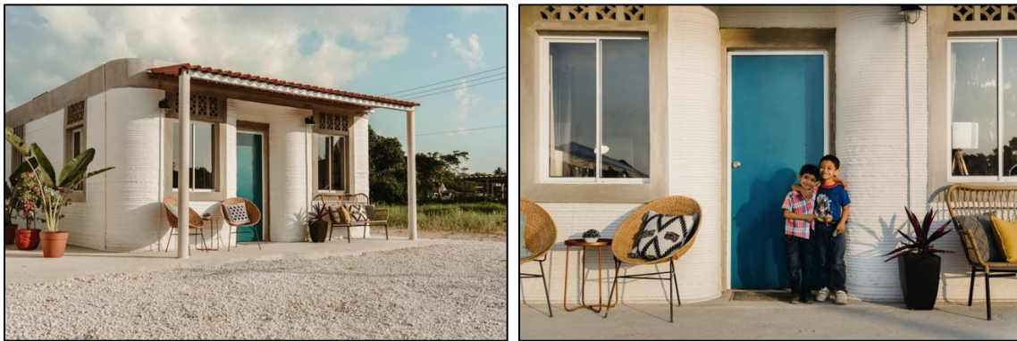
Figure 7. One of ICON’s initial two homes 3D-printed in Tabasco, Mexico [187].
