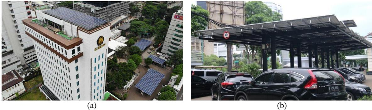
**Figure 7.** (a) Location of solar power plants of Setjen KESDM; (b) Installation method of solar power plants on the Setjen KESDM carport.
