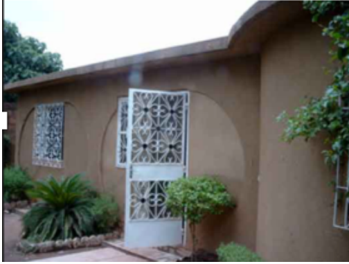
Figure 3.13: Medium income house Source: (Nko 'o, 2006)
