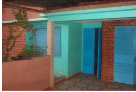
Figure 3.14: Example of medium income house Source: (Nko 'o, 2006)
