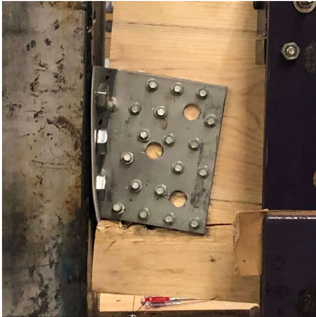
Figure 4.9: Connector rotation and fastener shear typical of shear deformation of AE 116
