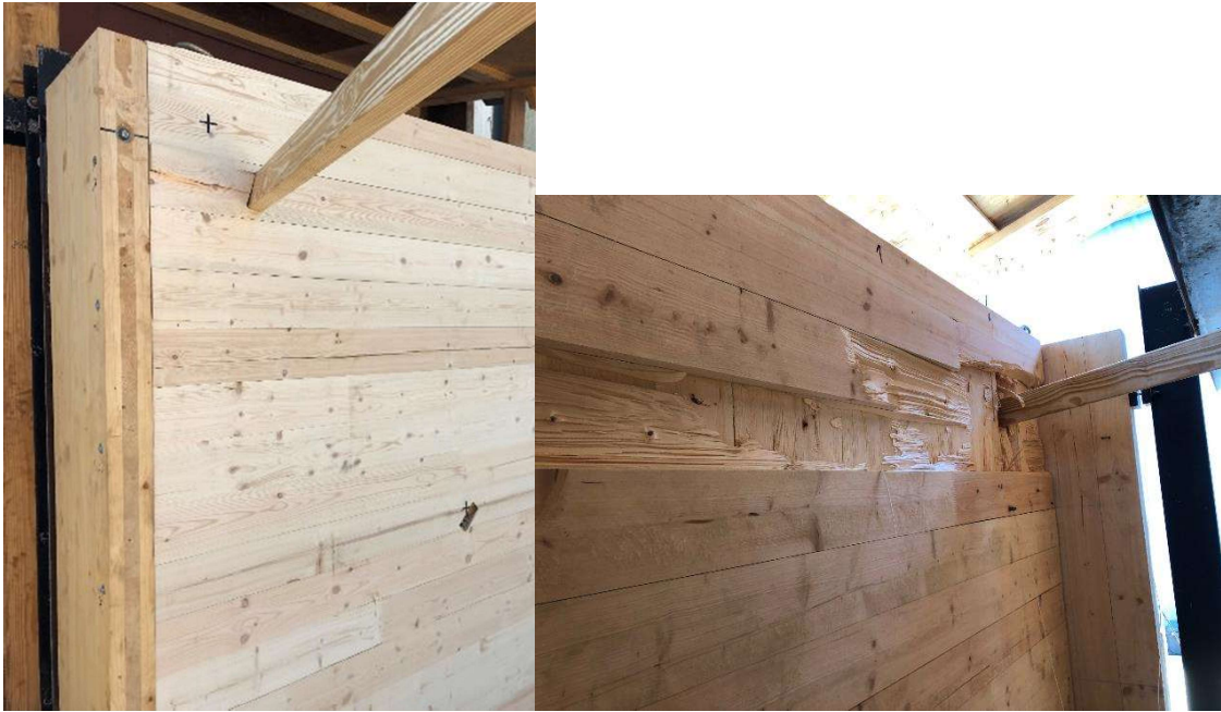
Figure A-30: Panel 10, strong-axis, weak-connection, corner, 15-pound, 112.7 mph, failed – perforation/dislodgement (front-left, back-right)
