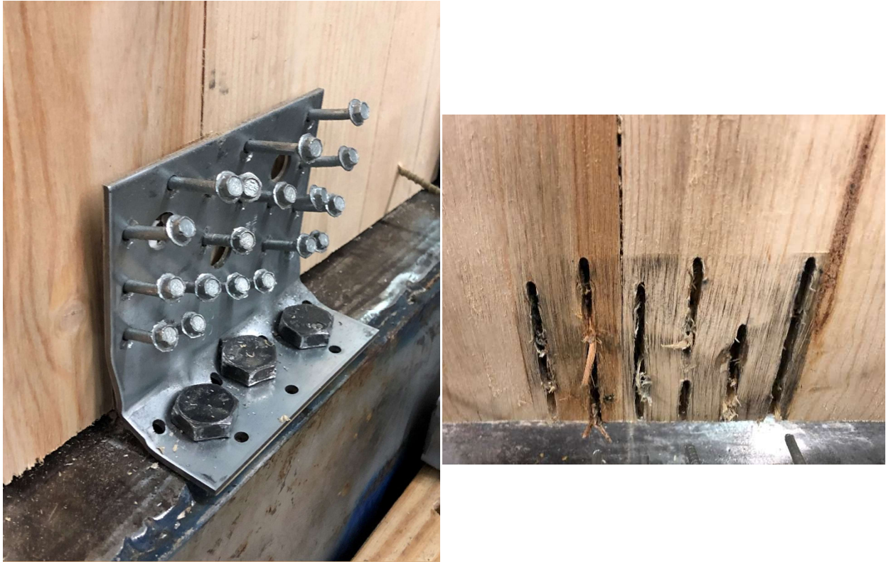
Figure 4.7: Cyclic uplift testing failure
