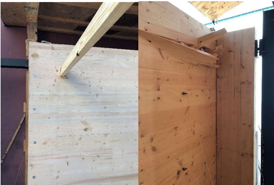
Figure A-33: Panel 11, strong-axis, strong-connection, corner, 9-pound, 103.9 mph, failed – permanent deflection (front-left, back-right)
