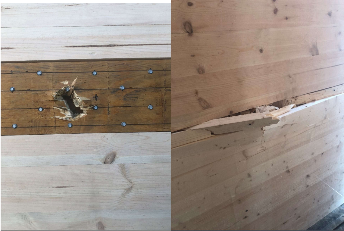
Figure A-46: Panel 18, strong-axis, surface-spline connection, center, 15-pound, 85 mph, passed (front-left, back-right)
