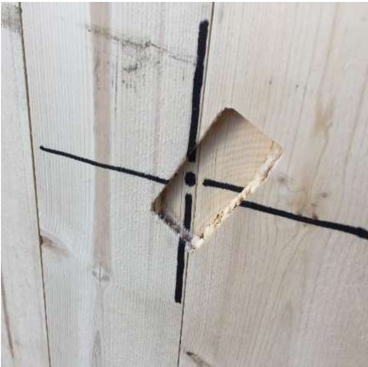
Figure A-1: Panel 1, weak-axis, strong-connection, center, 15-pound, 59.4 mph, passed test (front of panel)
