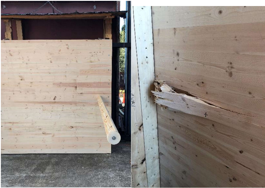
Figure A-32: Panel 11, strong-axis, strong-connection, edge, 9-pound, 105.8 mph, failed – permanent deflection (front-left, back-right)
