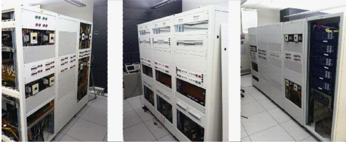
Figure 2-6. Photo of HTB Type I and Type III reconfiguration cabinet [27].
