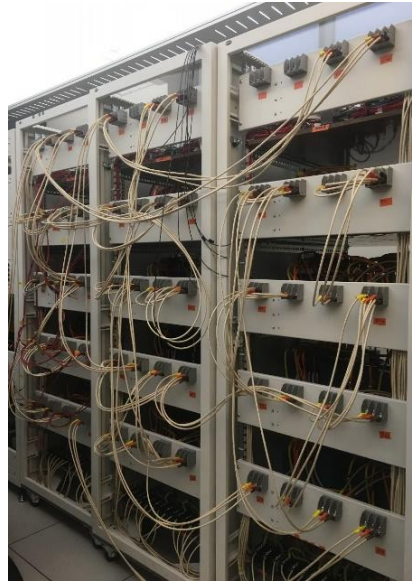
Figure 2-5. Photo of HTB Type II reconfiguration cabinet [27].
