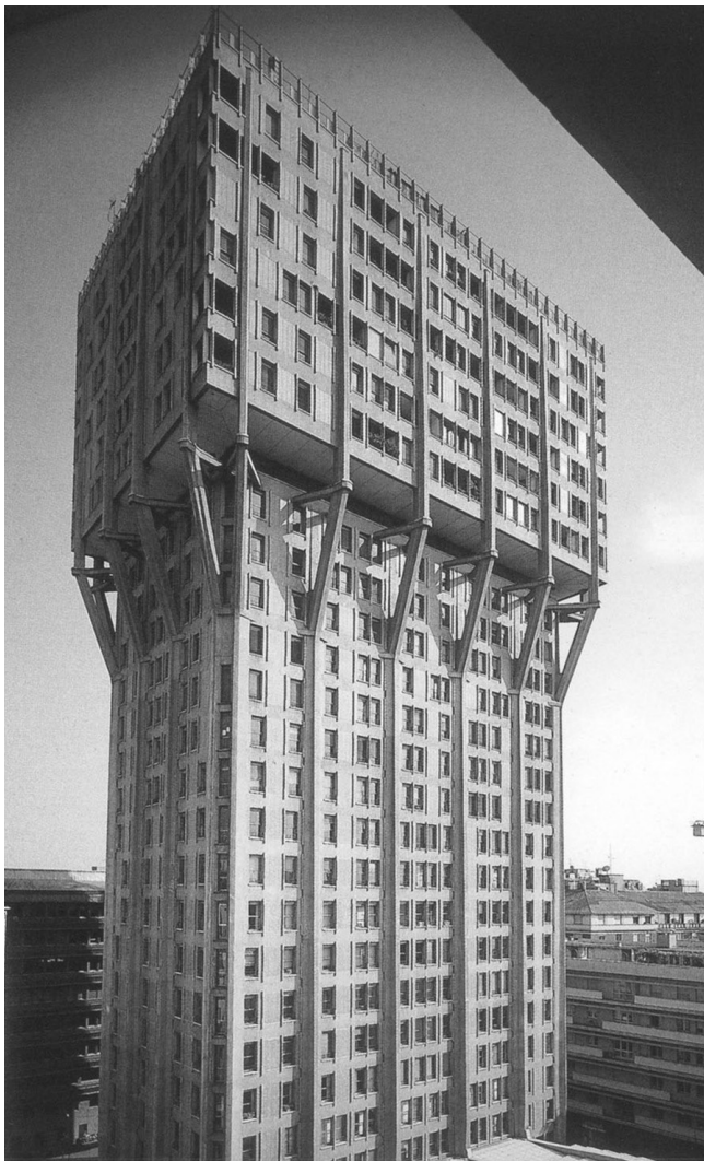
Figure 1. Velasca tower, Milan. General view.
