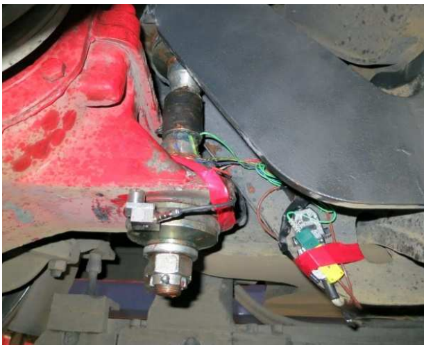
Fig. 11. Mounted and connected gearbox hinge [2]
