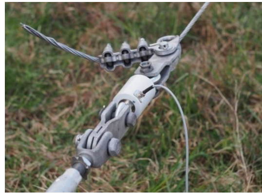
Fig. 6. Attaching of the load cell to sensing the axial force in conductor.
