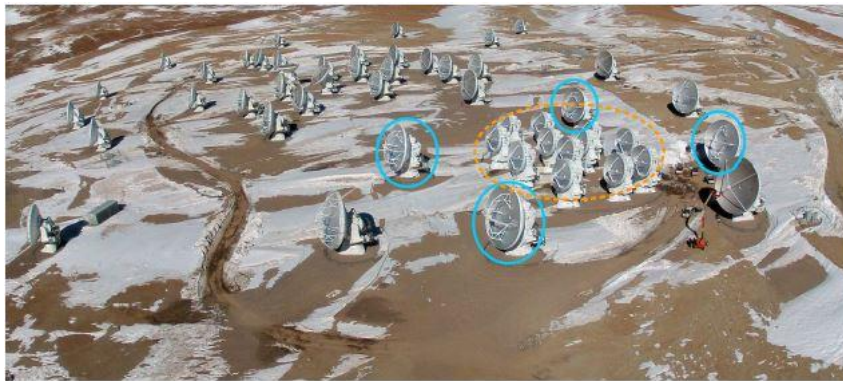
Figure 2.11. Picture of ALMA 12-m Array and ACA (Remijan et al., 2019). The ALMA 12-m array are distributed in left side of the image. ACA with all 7-m array antennas and four single-dish 12-m antennas are shown in dashed orange circles and blue circles, respectively.
