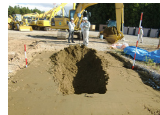
Fig.5 Excavation experiment using actual power shovel
