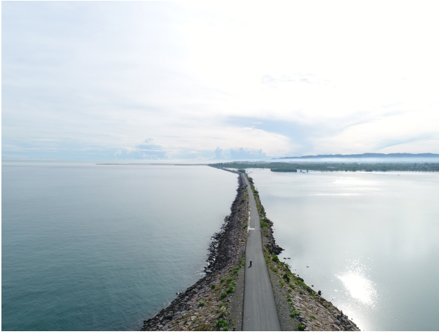
Figure 3. A 7 km embankment along the coast of Banda Aceh and a road which was constructed at its leeward side (date photo taken: February 2018).
