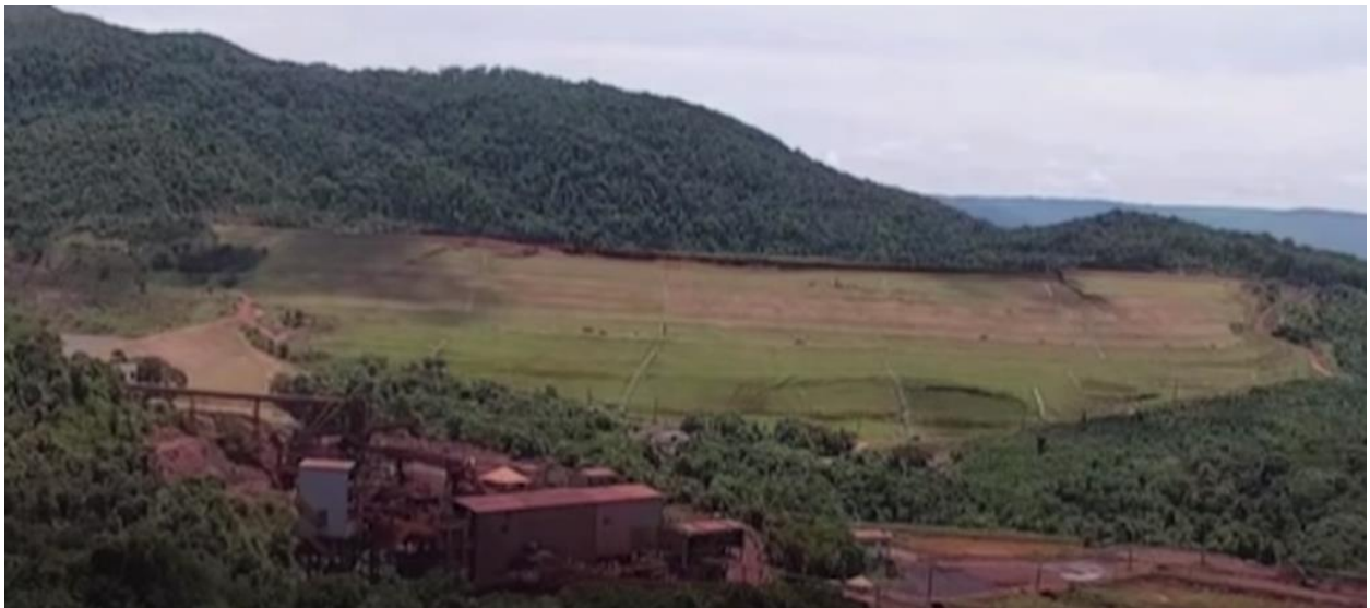
Figure 2 – Dam I when collapse started (Guardian News, 2019)
