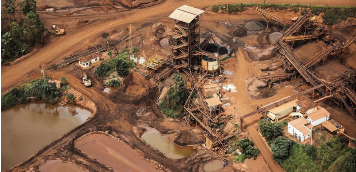
Figure 18 - Reparations to a plant after the incident (Darlington et al., 2019)
