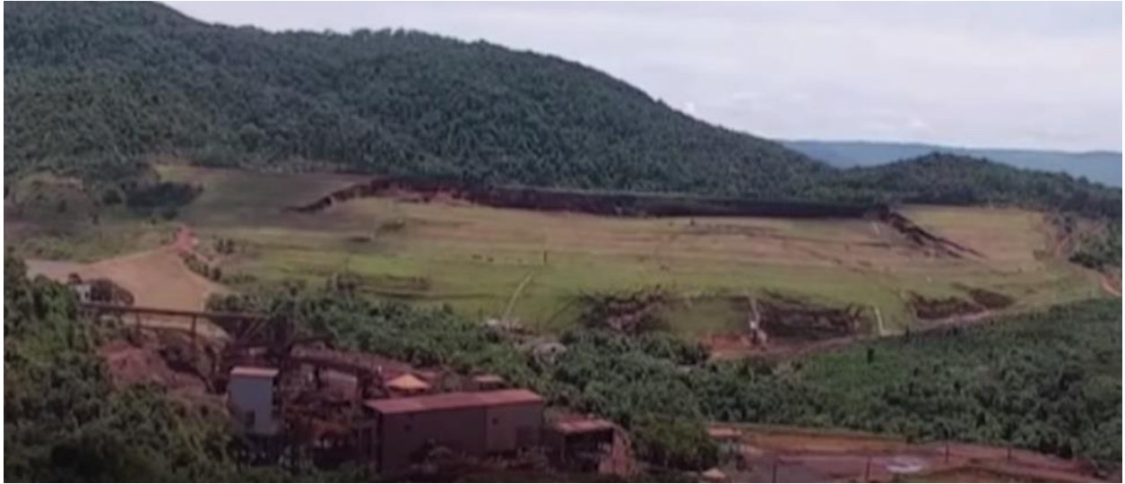
Figure 3 – A few seconds after the collapse started (Guardian News, 2019)
