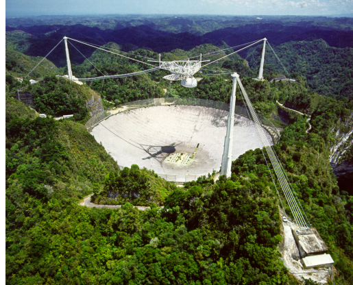
(b) The 300-m diameter Arecibo radio telescope in Puerto Rico, USA. Courtesy of the NAIC - Arecibo Observatory, a facility of the NSF.
