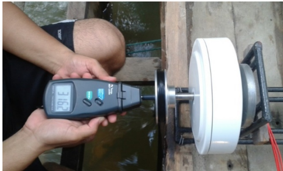
Figure 4. Shaft rotation measurements at the permanent magnet generator.
