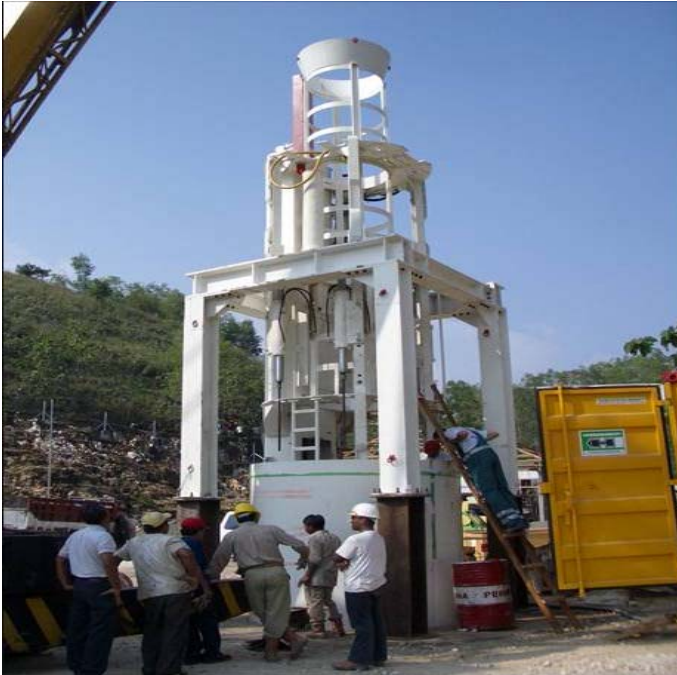
Figure 6 : Vertical drilling machine VSM 2500
