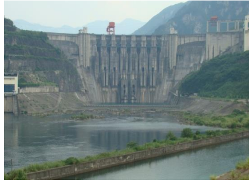
Figure 11: Dam of Hegeyan
