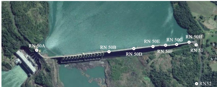
Figure 3: Approximate positions of the RRNN located on UHGJR dam.
