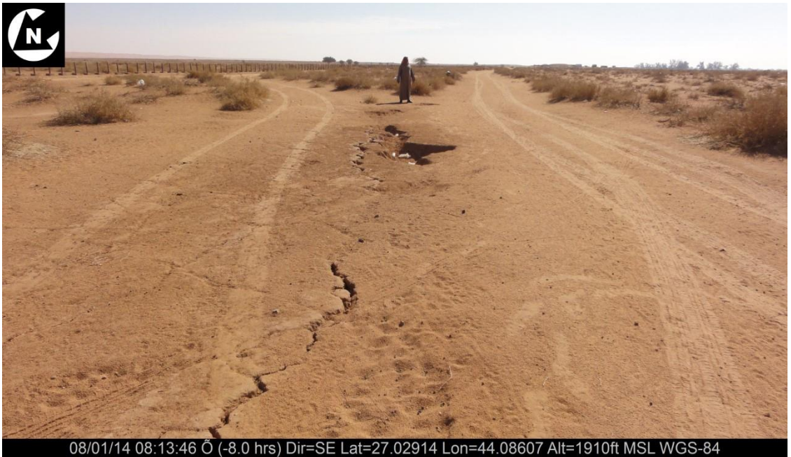
Figure 3.6 Some types of cracks and fissure at the Turubah city areas.
