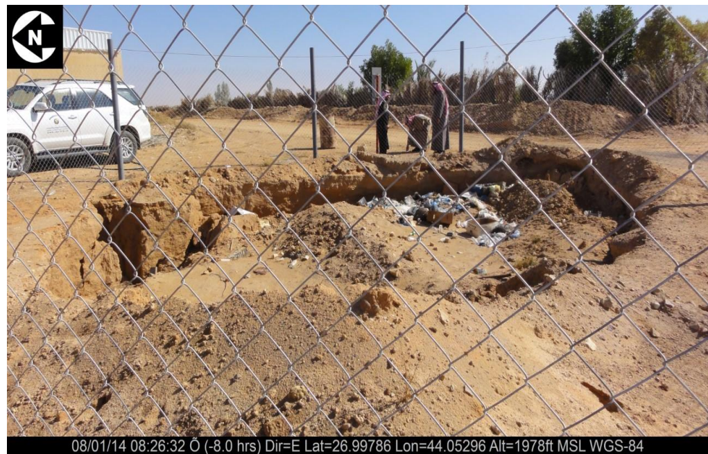
Figure 3.7 Sinkhole at the studies areas.
