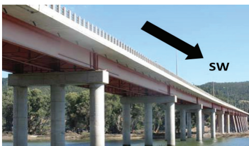
Fig. 1. Partial view of the bridge structure
