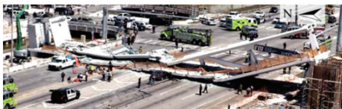
Fig. 2. Collapse scene of the pedestrian bridge
