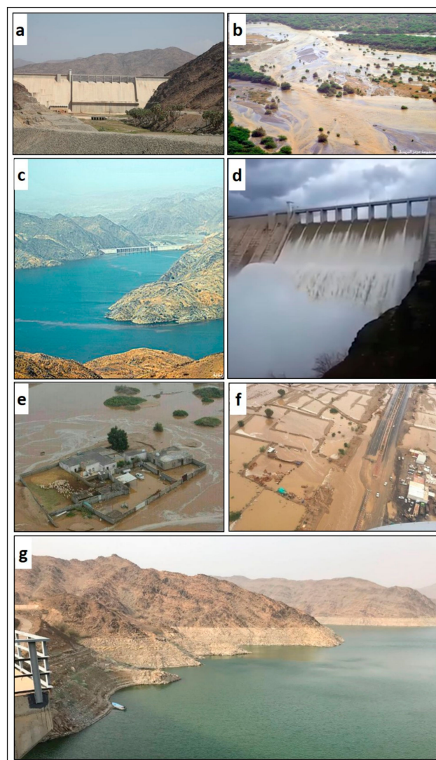
Figure 2. Photographs showing; (a) dam is concrete, (b) inundation of agriculture areas during the flood, (c) reservoir capacity reaching the spillway, (d) water flow over the spillway, (e) flood water invading the villages, (f) floods rendering the roads and highways impassible, and (g) water level change in the reservoir due to continuous discharge of water from reservoir (according to the KSA authority request).
