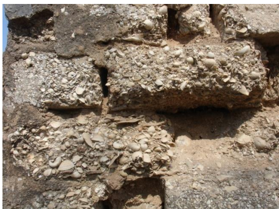
Fig. 3. Arca layer with placura placenta was cut into bricks for construction of house walls by Nghe An people [Source: Cao Dinh Trieu (2011)]
