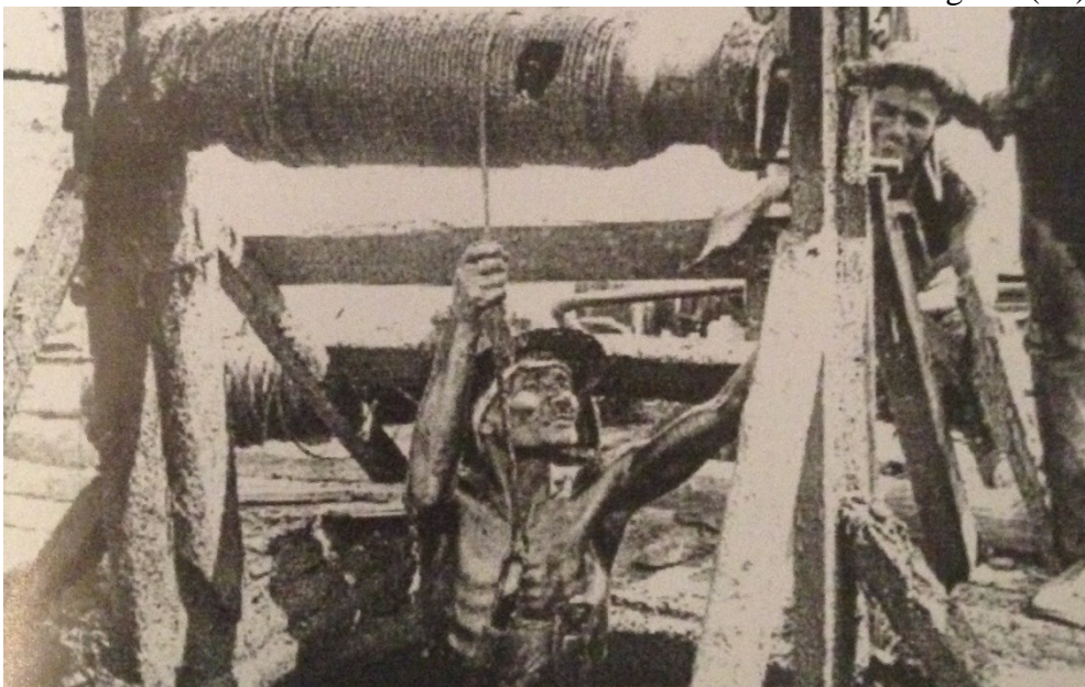
Oil well drilling in XIX century in Baku
