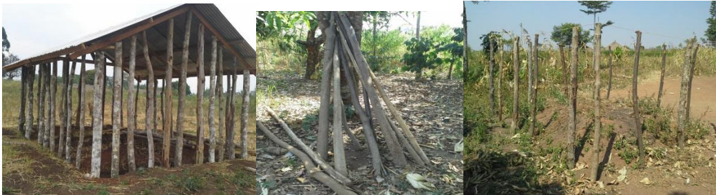
Figure 4: Poles extracted for construction
