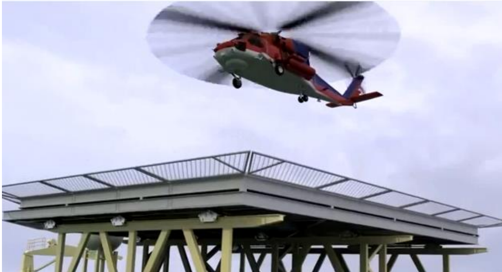
Figure 10.13: Screenshot from an animation video where a helicopter is approaching the ARC helideck which can move about \pm 2.60 meters back and forth on the skids (Uptime International AS, 2010)
