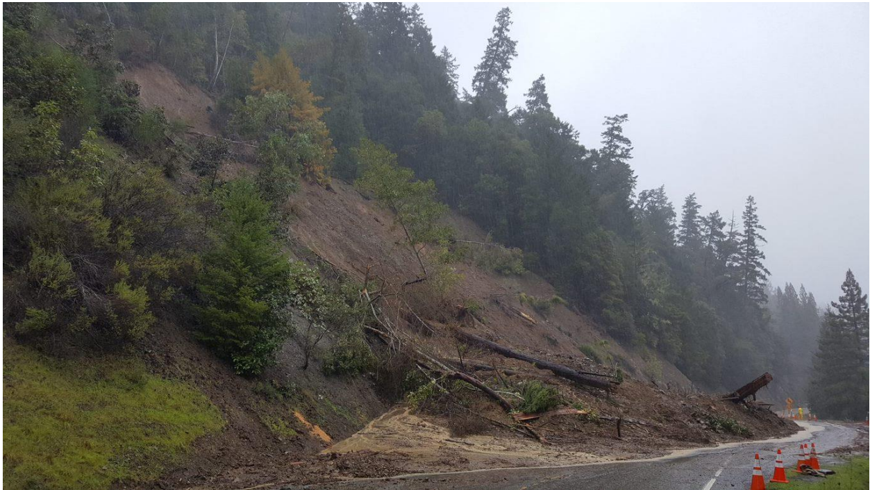
FIGURE 10-2: SR 1 NEAR LEGGETT MUDSLIDE
