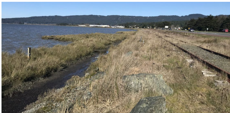
Figure 5. Existing dike (as a railroad grade) near proposed Indianola Interchange.
