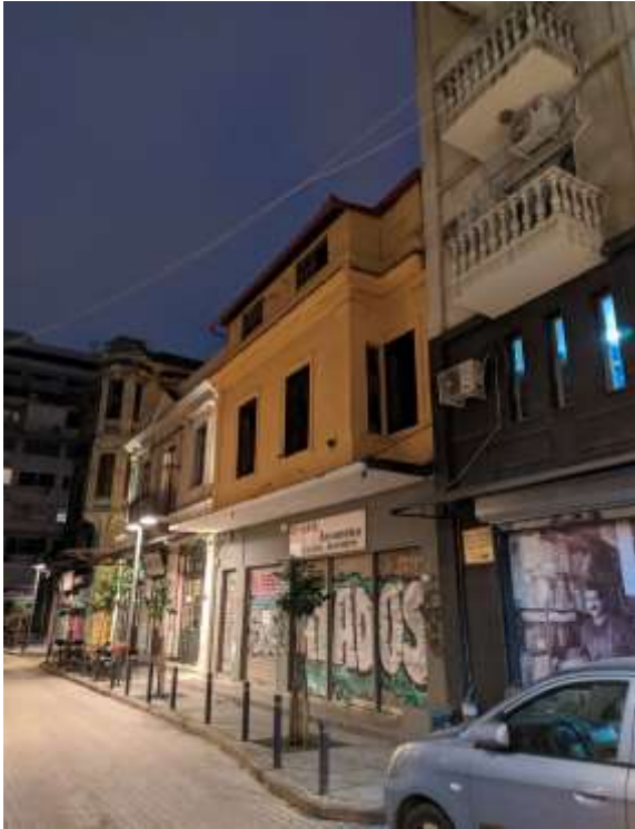
Figure 1 Photo of the building at 7 Edessis Street, author photo.
