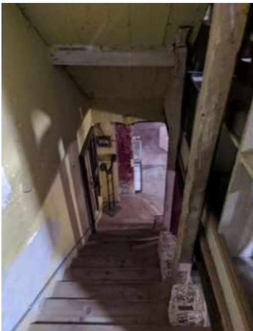
Figure 8 Staircase leading to basement, author photo.
