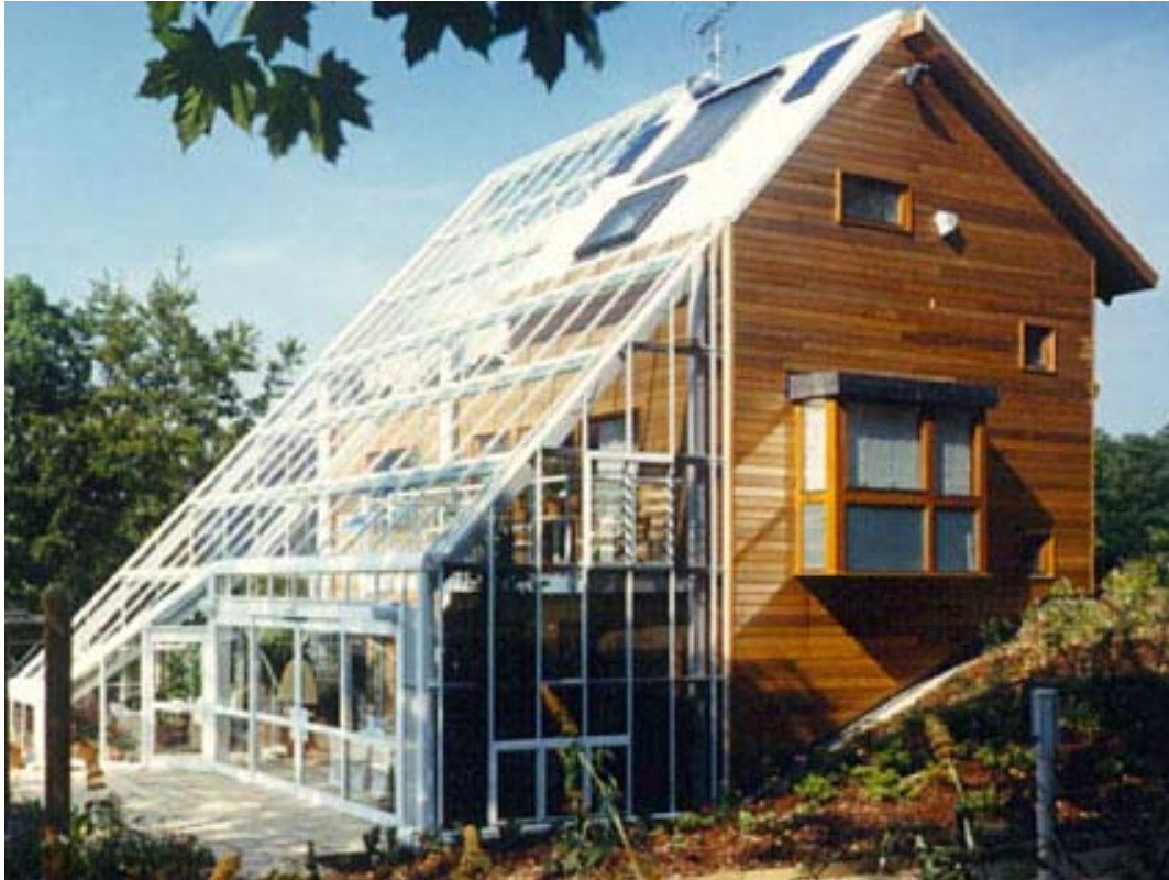
Figure 6. Integer Millennium House built at Watford in 1997. The house was built according to the passive solar design principles including a wedge shaped south facing attached sunspace.
