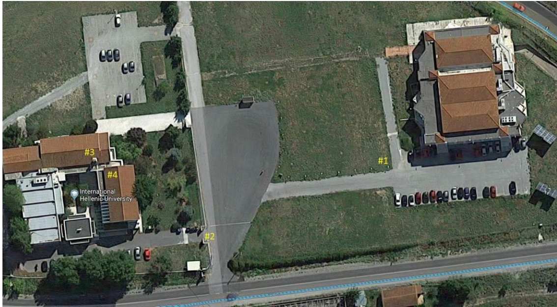
Picture 11: Node placement as seen from above (IHU campus)
