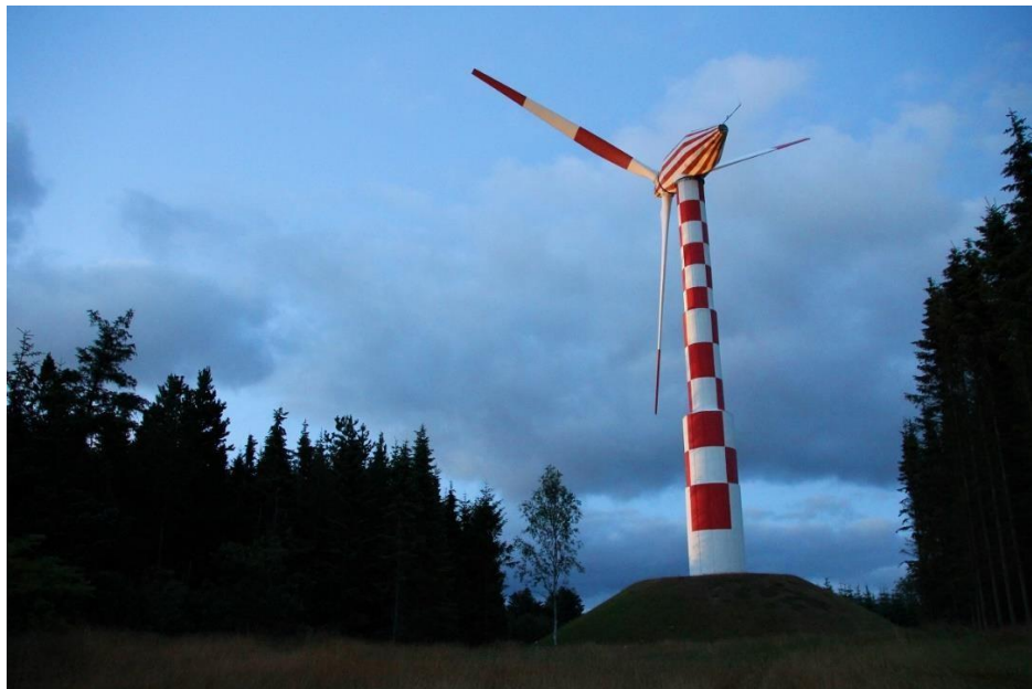
Figure 17 First TVIND Wind Turbine 20
