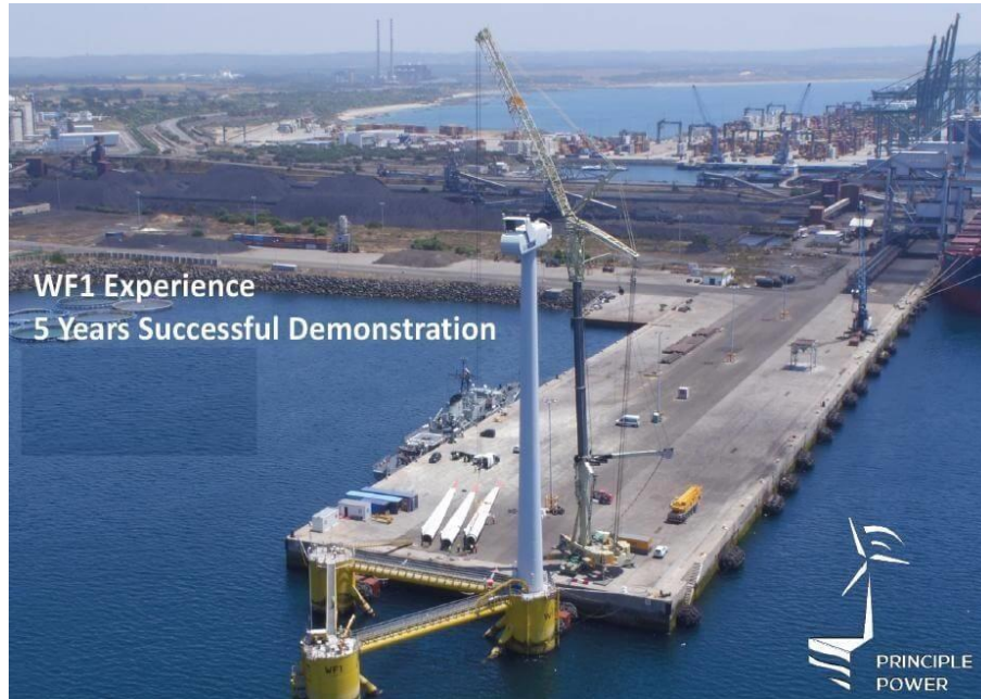
Figure 81 The WindFloat rests at dockside during its recent decommissioning in Portugal. It was deployed in 43 m of water and came online in 2011 88
