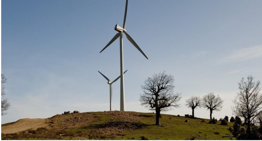
Figure 129 Kafireas Enel Greenpower's project 136
