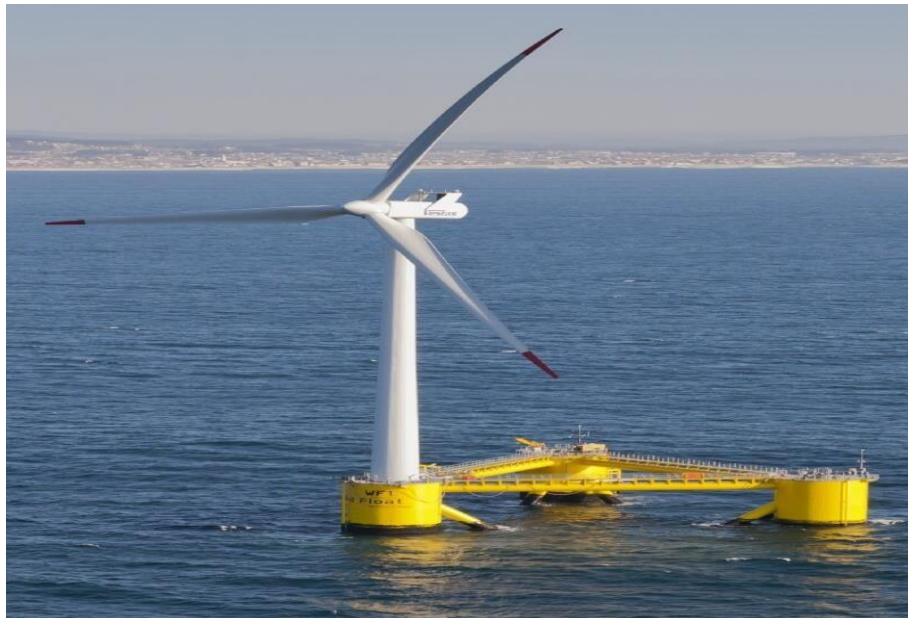
Figure 82 The WindFloat during its sea trials was anchored off the coast of Portugal 89
