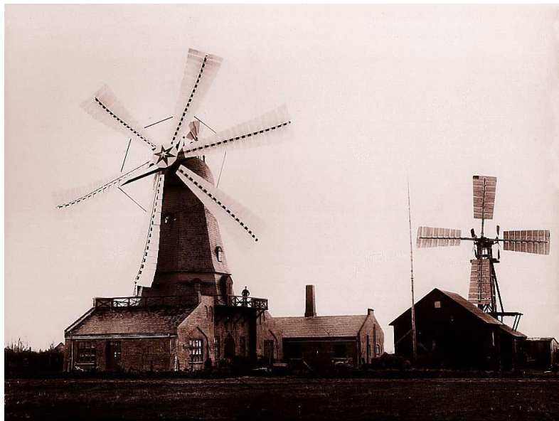
Figure 11 P. la Cour's electricity generating WT that is utilized to cover the lighting of Askov 14
