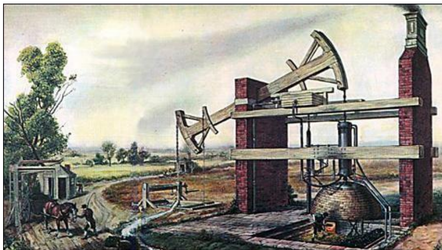
Figure 2 Upgraded steam engine by T.Newcomen (1712) 2
