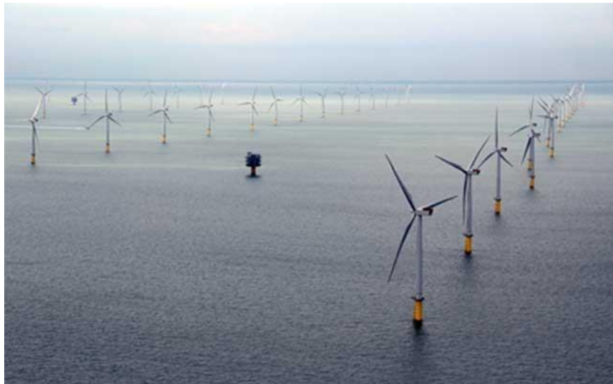
Figure 23 London Array WF. 175 turbines of 630 MW Round 2 offshore wind farm is located 20 km off the Kent coast in the outer Thames Estuary in the United Kingdom 26
