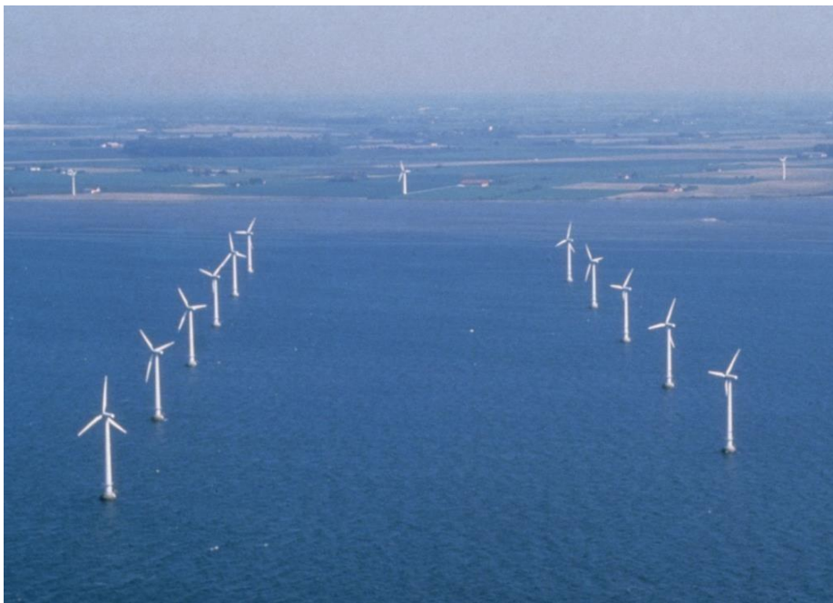
Figure 18 First Offshore Wind Farm (Vindeby), 4.95MW, built in the Danish Baltic Sea, near the island of Lolland, in 1991. 21
