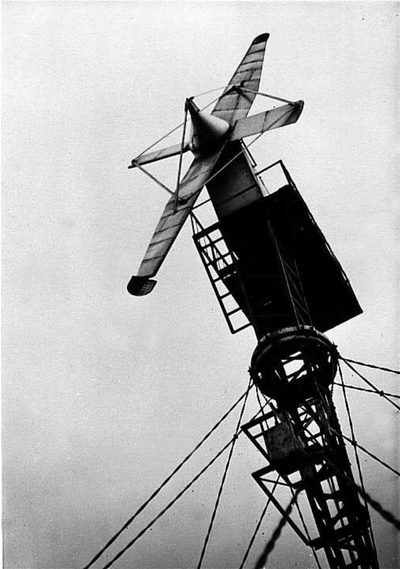
Figure 16 First AC wind turbine by J.Juul 19
