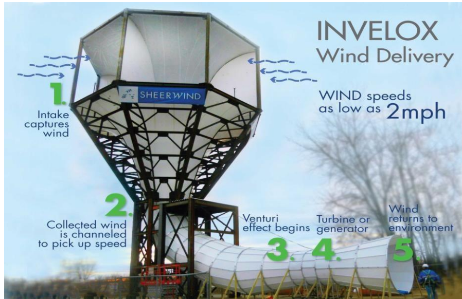
Figure 121 SheerWind Invelox windtube, the steps of the process 128
