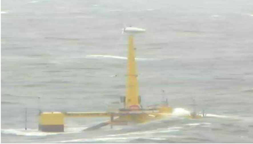
Figure 83 Team Dagher’s proof of concept mounted a 20-kW turbine on a floating concrete platform. The initial project was a 1:8 scale of a 6 MW floating turbine launched in the Gulf of Maine in 2013. The next project will be a modest farm of two 6-MW floating turbines anchored about 14 miles off the coast of Maine near Monhegan Island, for which the DOE provided a $39.9 Million grant. 90
