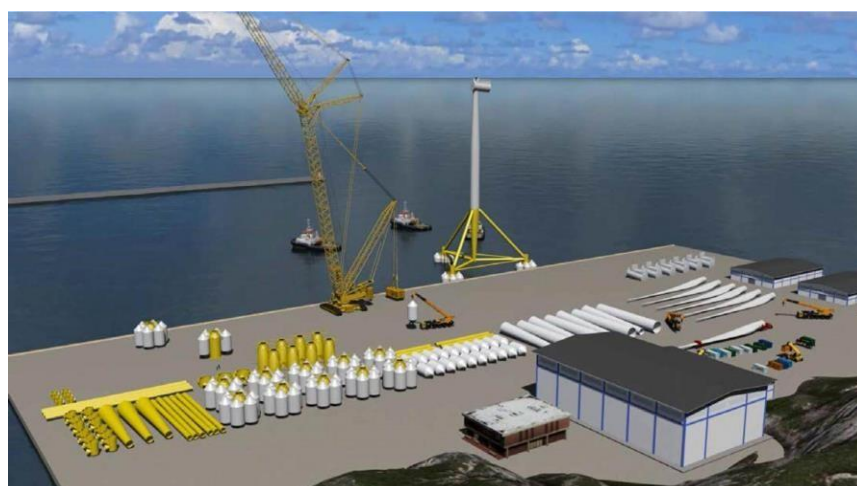
Figure 86 TetraSpar foundation 93
