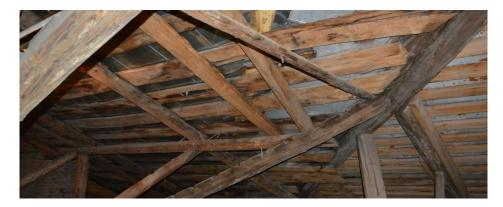
Fig. 5. Attic. The state of the truss system and roof **Analysis. Preliminary engineering opinion.**
