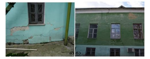
Fig.4. The courtyard facade: a - condition of the lower part of the wall of the extension of the end of the 19th century;
