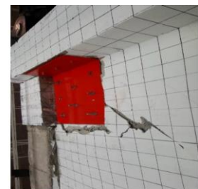
(f) corner failure
