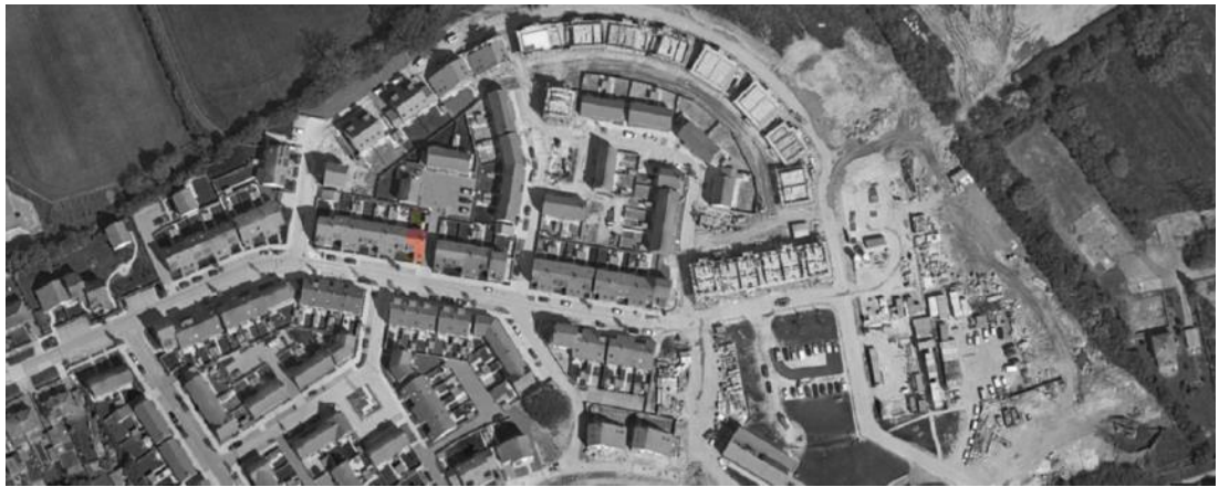
Fig. 5.14 Aerial view of development where house UK54 is located in York
