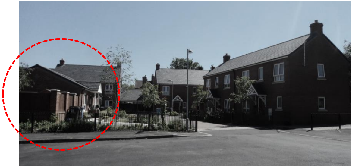
Fig. 5.11 Passivhaus development where UK52 is located
