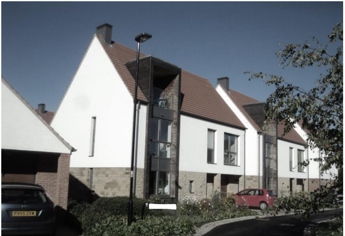
Fig. 5.19 East street façade view of UK55
