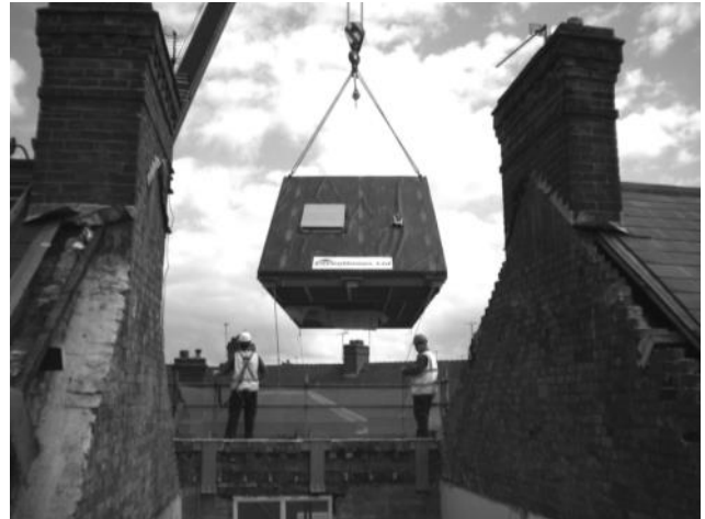
Fig. 5.7 Roof pod installation on-site
