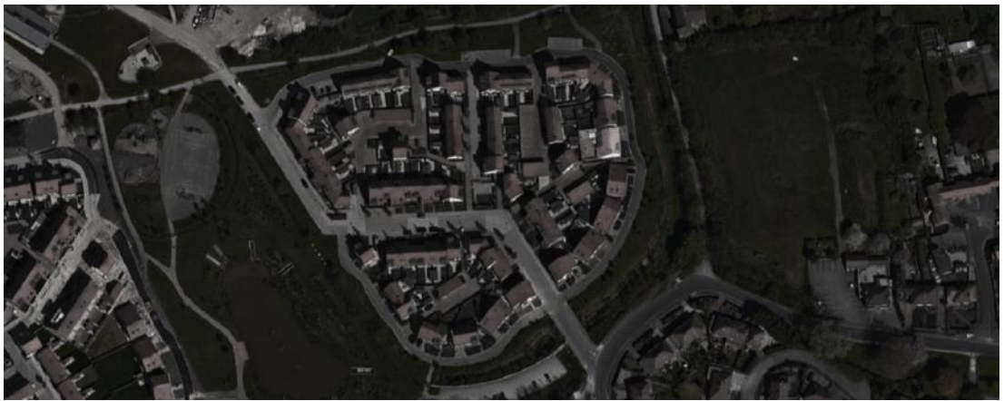
Fig. 5.18 Aerial view of development where house UK55 is located in York
