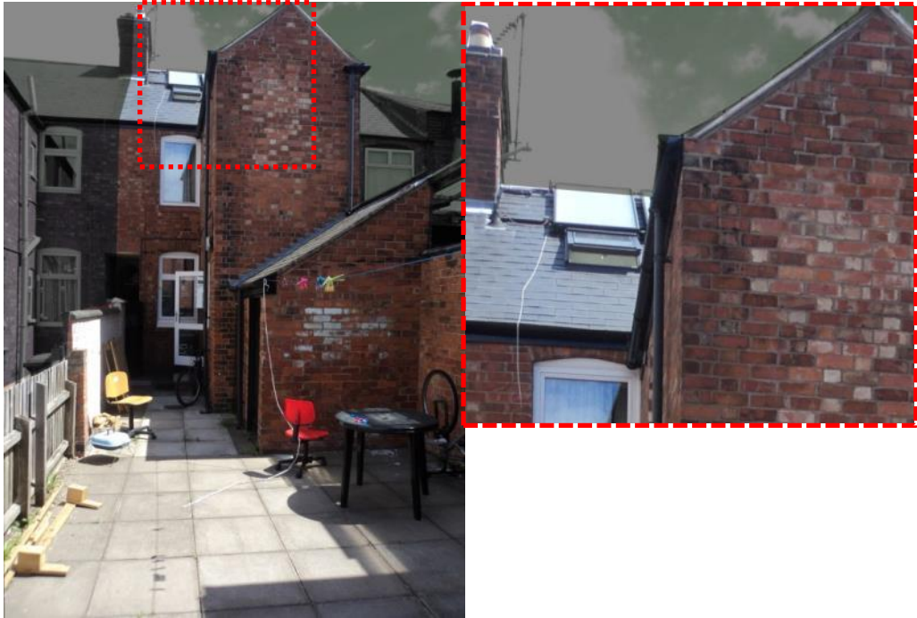
Fig. 5.8 UK51 solar thermal: rear (left) and detail (right)
