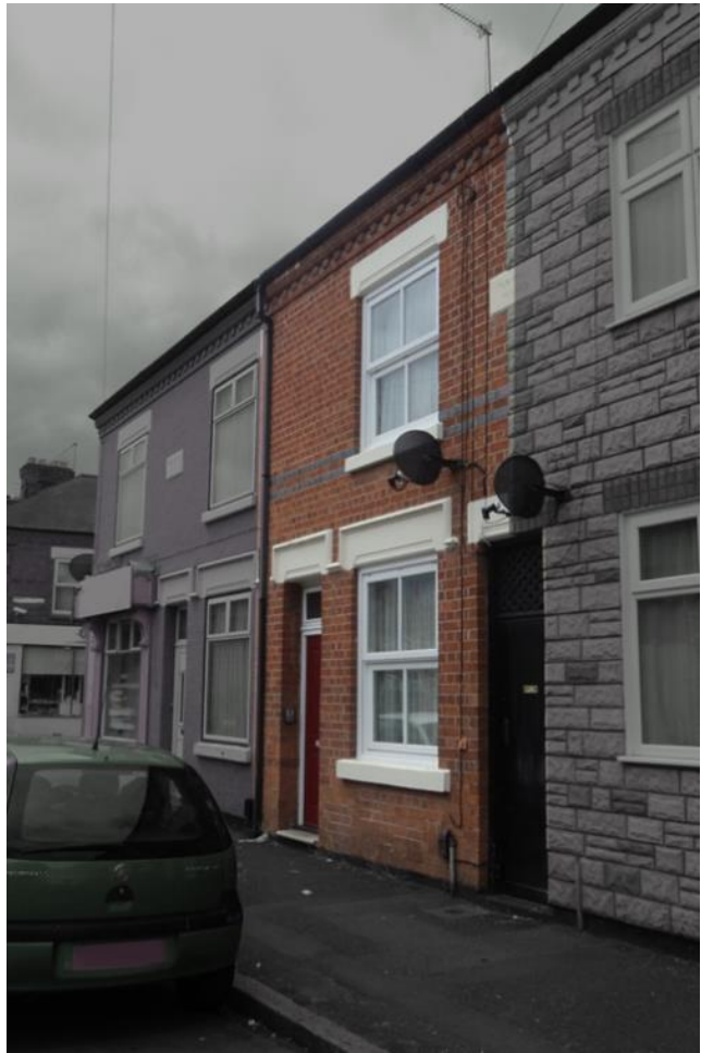
Fig. 5.2 East façade view of the Victorian terrace (late 19 th century) retrofitted to Passivhaus-like standards UK51
