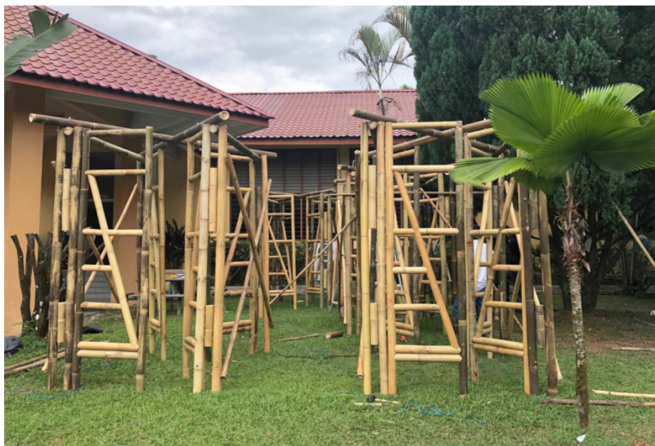
Figure 2. Bamboo Pavilion Structure. Authors, 2019.
