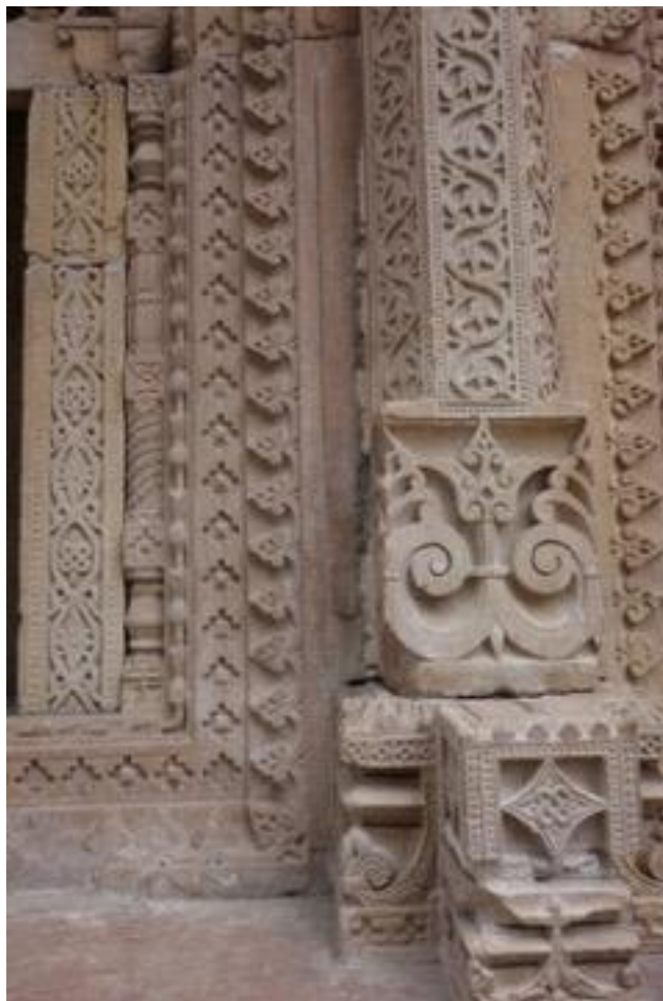
Figure 15. Detail of the wall of the Jama Masjid in Chanderi
