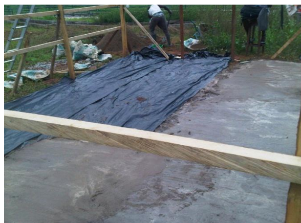
Figure 1: The Greenhouse floor at the DPC level
