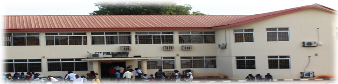
Figure 5.29 A building project on-campus sponsored by ETF in 2002 for offices and laboratories
