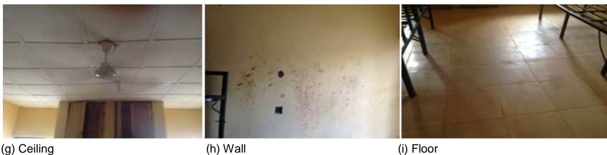
Figure 5. 48 Conditions of a typical bedroom at Case C1
