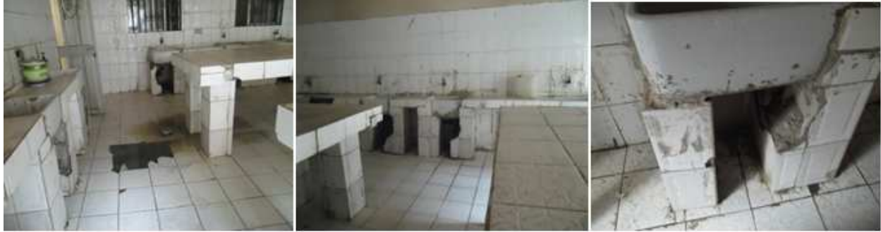
Figure 5.36 A laundry room in a hostel block at Case B3
