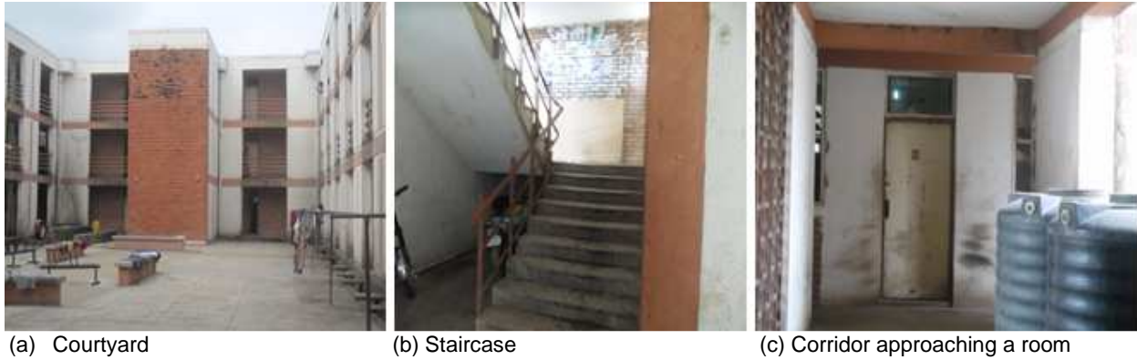
Figure 5.17 Interior Views at Case A3
