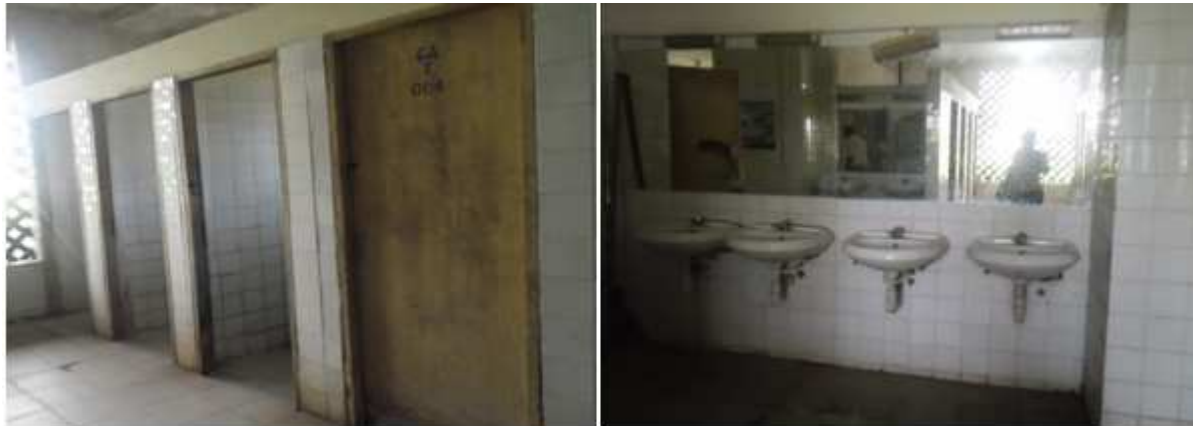
Figure 5.7 A lavatory area in the female hostel block at Case A1
