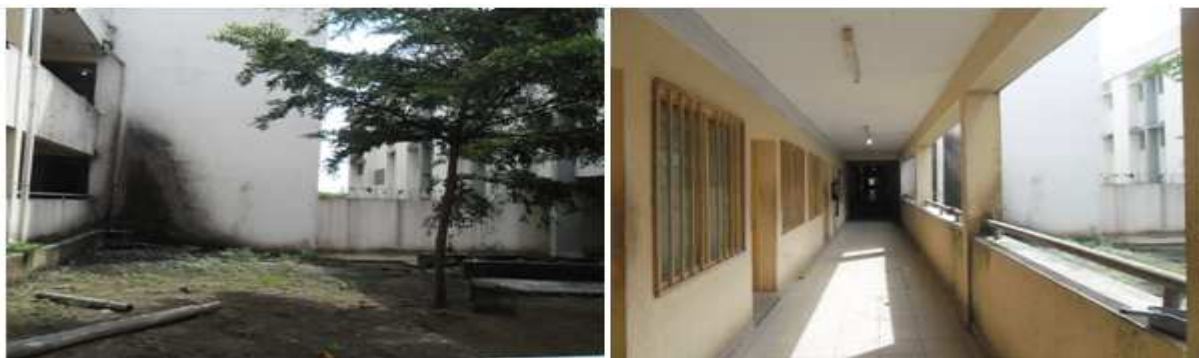
Figure 5.4 Views of the courtyard and a corridor at the female hostel block at Case A1
