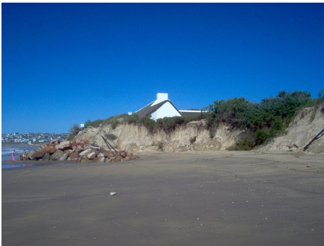
Figure 1.4 Photograph taken 20 March 2007, showing increased erosion adjacent to revetments and behind the end of revetment, known as “end effect” or “flanking effect”.
