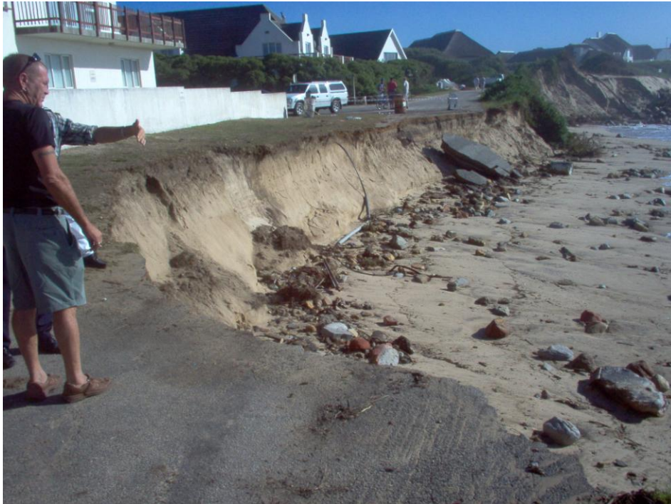
Figure 4.16 photograph taken at 10 am, 20 March 2007, a 40 m section of Ralph road was totally undermined and erosion cam with 2m of the property behind (Picture by Author).
