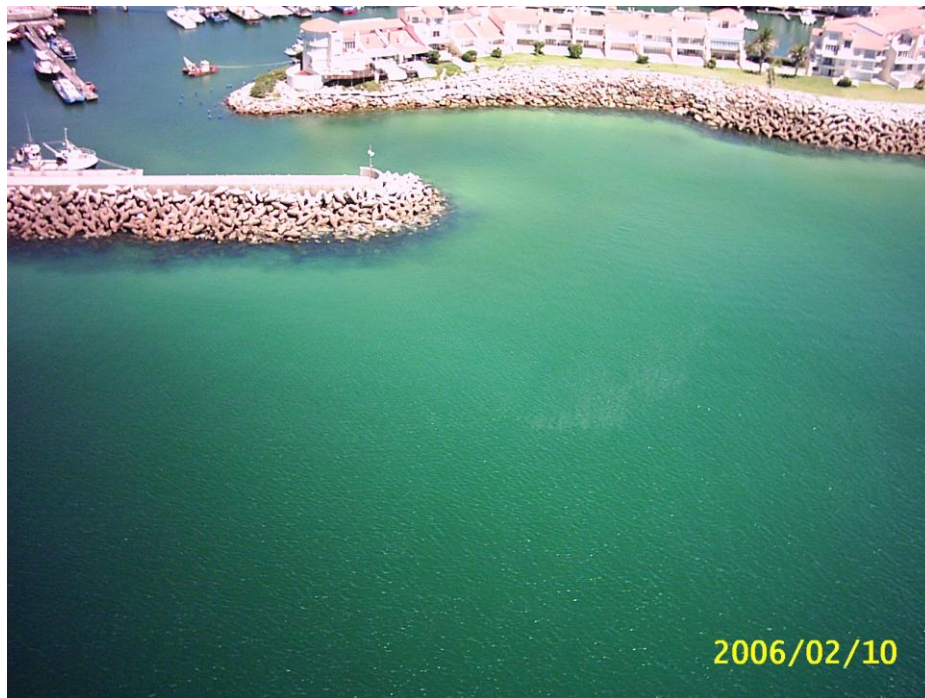
Figure 4.7 Oblique aerial photograph of Port St Francis and close offshore, seabed is completely sandy, with no reef visible.
