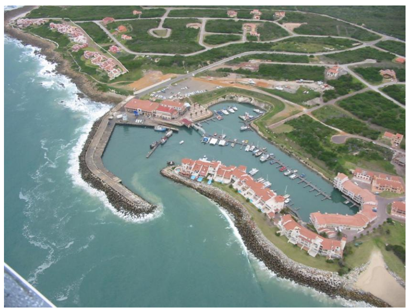
Figure 5.10 Port St Francis acts as a substantial interruption to longshore currents along the Cape St Francis Headland.
