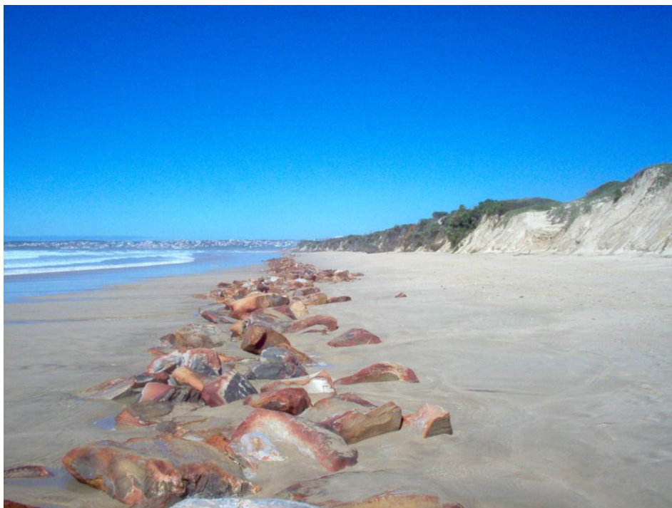
Figure 4.17 photograph taken 10:30 am, 20 March 2007, large volumes of sediment were eroded from the dune areas along the artificial barrier dune, this storm exposed an old line of revetment which had sunk and been buried (picture by the author).
