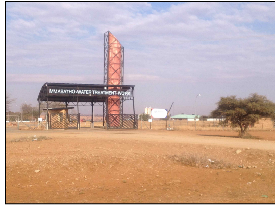
The Mmabatho Water Treatment works to the west of Mahikeng. This plant treats water from the Setumo Dam.
