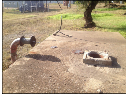
One of the public water supply boreholes at Grootfontein, abandoned due to falling groundwater levels.
