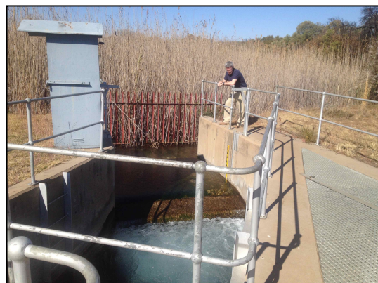
The weir measuring the natural discharge of the Molopo Eye.
