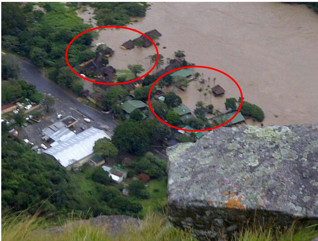
Figure 6.4: Flooded Port St Johns resorts along the Umvimvubo River
