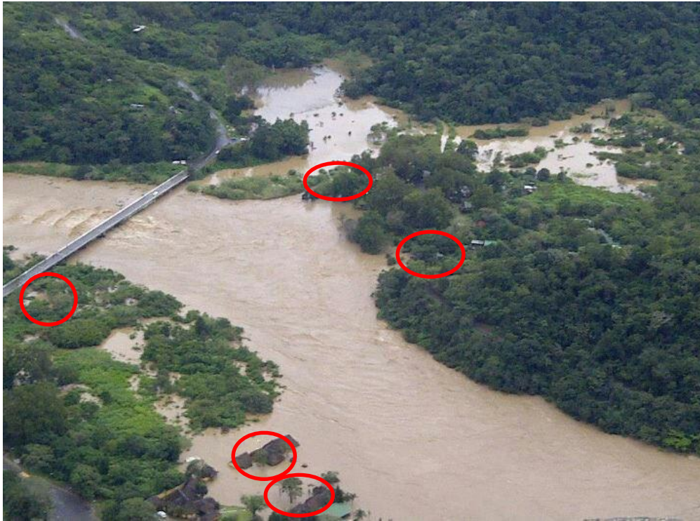
Figure 6.3: Flooded Umvimvubo River and submerged resorts.
