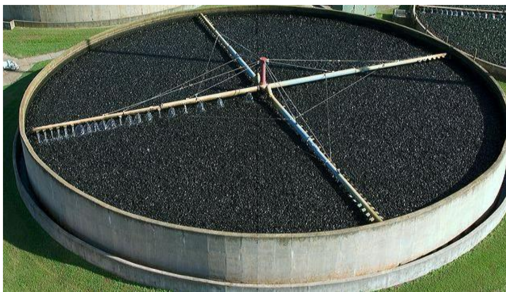
Figure 2.6: Trickling filter wastewater treatment plant (www.igreenion.com).
