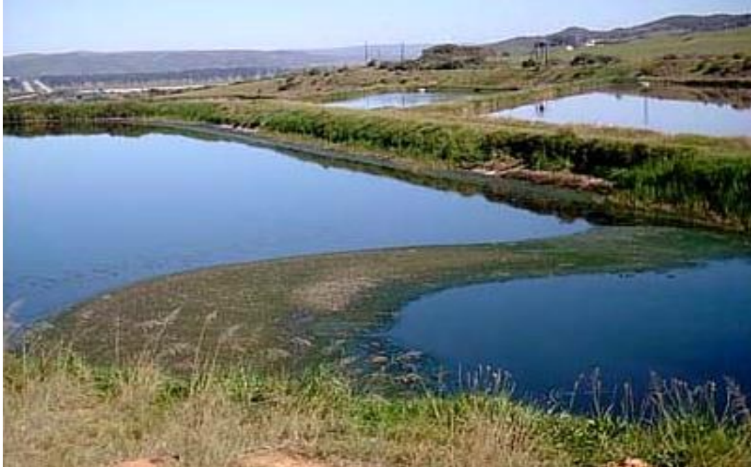
Figure 2.3: Oxidation ponds with different facultative and stabilization ponds ( www.biosystemssa.co.za ).
