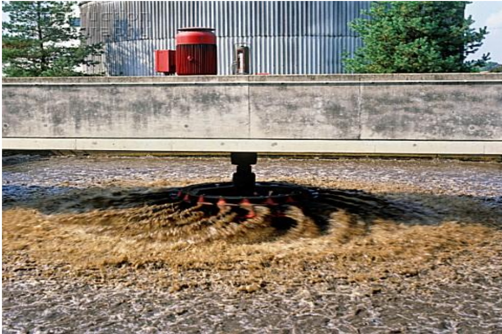
Figure 2.4: Activated sludge wastewater treatment technology ( www.constructionphotography.com ).
