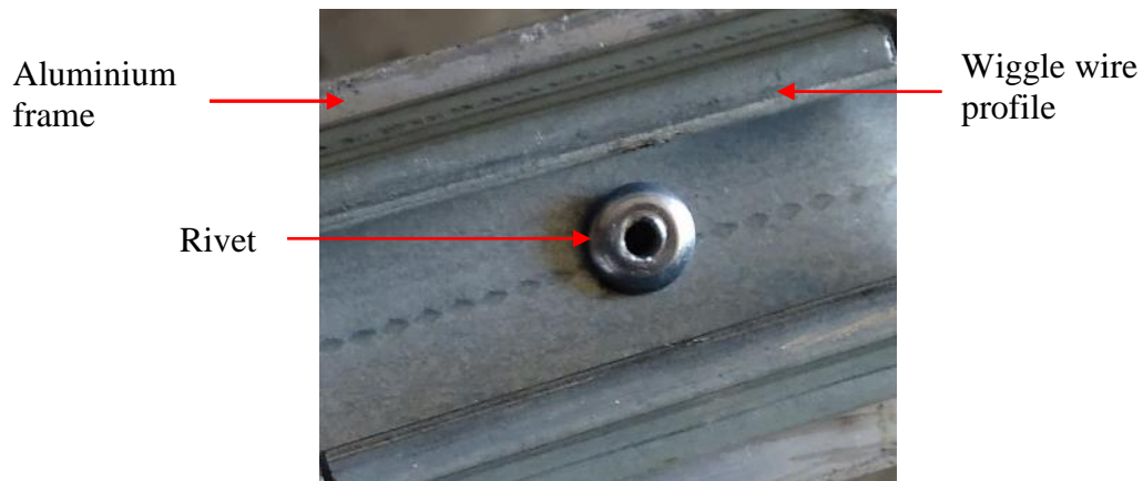
Figure 4.14: Riveted wiggle wire profile
