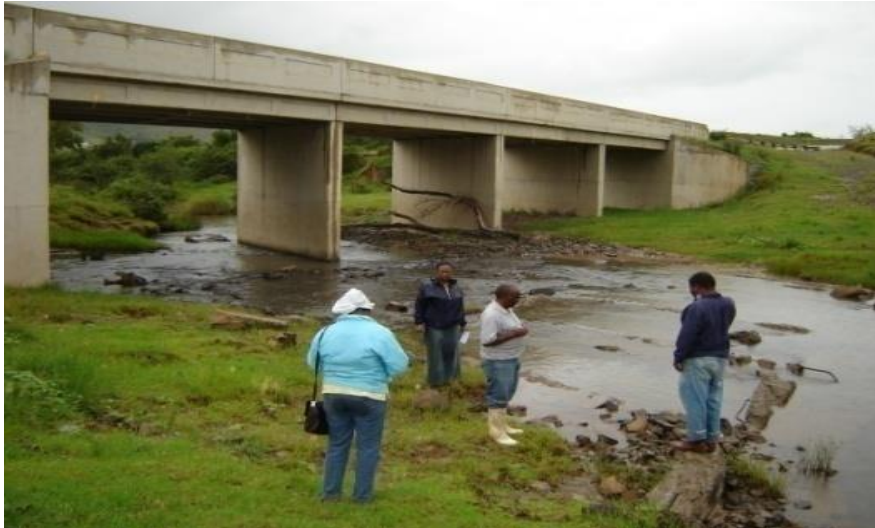
Fig. 2.8 Study Site 7: Gqumashe (32° 45' 477" S, 26° 51' 98" E) showing anthropogenic influence evident by a modern bridge
