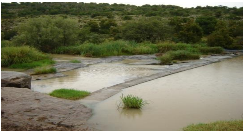
Fig. 2.10 Study Site 9: Njwaxa (32° 52' 538" S, 26° 53' 531" E) showing a ridge of Cemented dam across the entire width of the river
