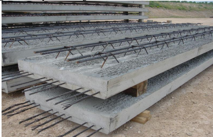
Figure 4. Reinforced concrete beams placed at the construction site in Baghdad Iraq [6]
