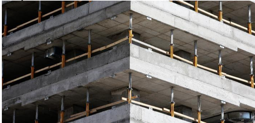
Figure 2. Reinforced concrete beams-based building under-construction in Basra Iraq [5]
