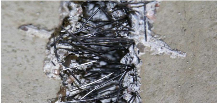
Figure 3. Highly promising materials for retrofitting purpose are the reinforced concrete (RC) composites [5]
