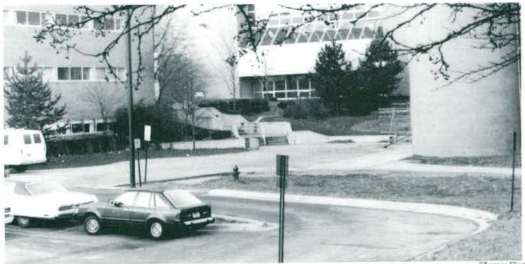
The Warren Olds building, called the REC/IM by students, received new additions this year enhancing students' workouts
