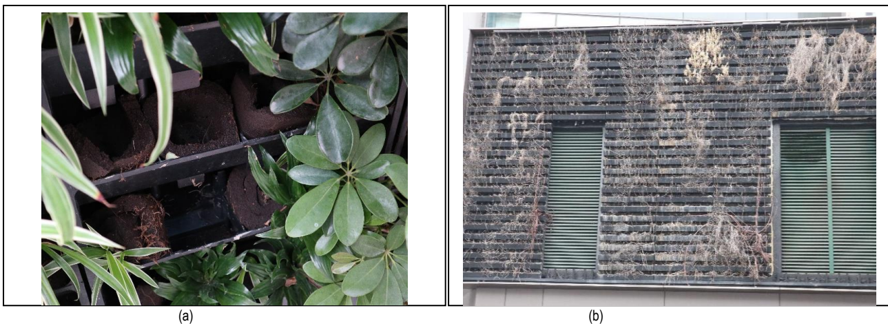
Fig. 2. (a) Hydroponic sponge as a soilless medium is widely adopted in LWS of Hong Kong. (b) Plant failure is found more common among outdoor LWS which rather dependent on a robust irrigation system.
