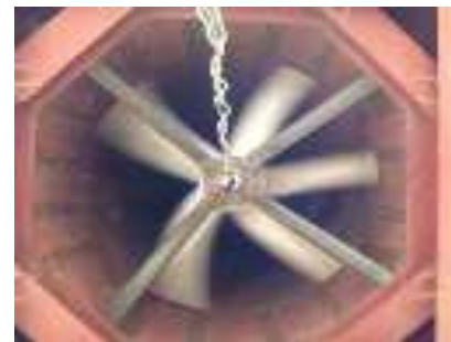
(b) Inside the chimney
