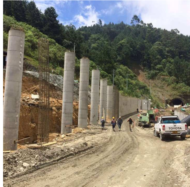
Figure 6. Works attached to the tunnel (Icconstructores, 2017).
