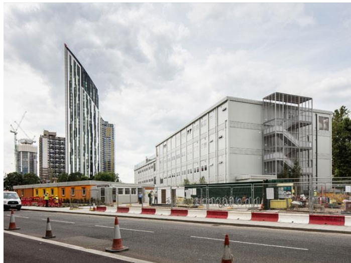
Figure 3: Temporary Modular Building – aesthetically pleasant (Wernick, 2017b)
