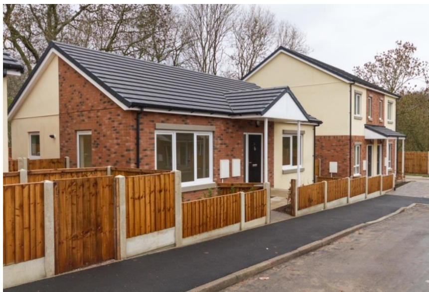
Figure 2 Completed Modular build development
