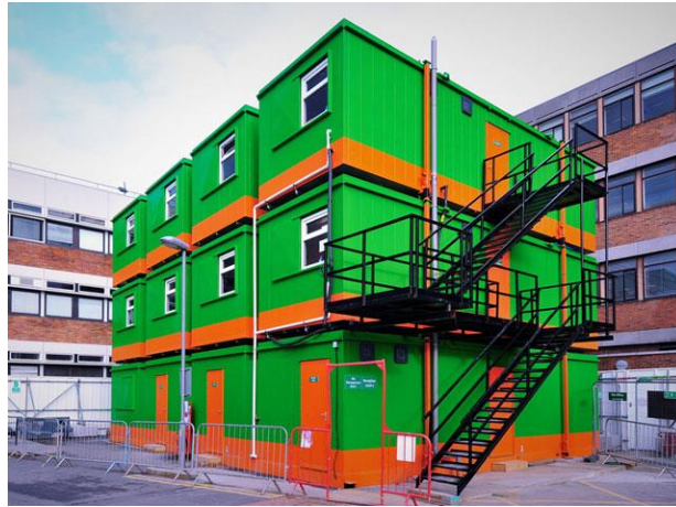
Figure 2: Temporary Modular Building – aesthetically non-pleasant (Wernick, 2017a)
